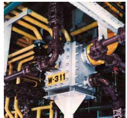
Compabloc asymmetric multipass condenser makes condensation and subcooling possible in the same unit
