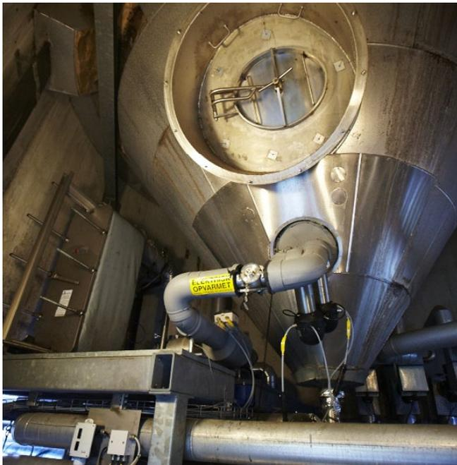
The Iso-Mix system installed in Carlsberg's fermentation tanks include a plate type heat exchanger, which enables much faster cooling.
